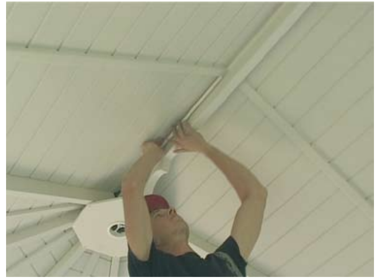
Roof seam strips are mounted with 4 nails/strip and after stiffening strips inner corner strips are attached (after sealing of the bushings) with 38 mm dyckert nails, 5/corner). The roof seam strips have left- and right-handed miter cuts. 2 + 2 short seam strips come between the ridge beam and roof elements, in Oval special roof elements 2 + 2 longer seam strips, left and right miter cut.
