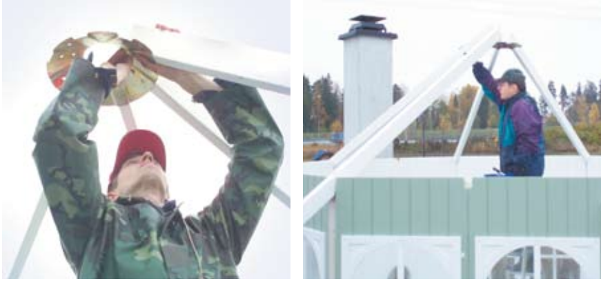
Picture of steel connecting plate above and beside, picture of plywood attachment used in hexagonal in the two above.
