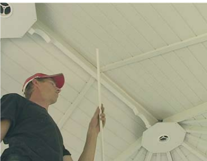
Roof seam strips are mounted with 4 nails/strip and after stiffening strips inner corner strips are attached (after sealing of the bushings) with 38 mm dyckert nails, 5/corner). The roof seam strips have left- and right-handed miter cuts. 2 + 2 short seam strips come between the ridge beam and roof elements, in Oval special roof elements 2 + 2 longer seam strips, left and right miter cut.
